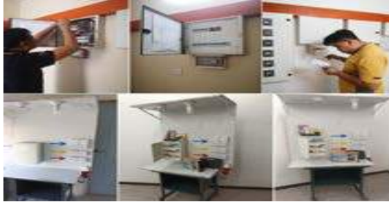
Figure 2. IoT Electrical Energy Audit Lab Kit produced for Energy Management System and Energy Auditing (DEQ40023) practical session.
